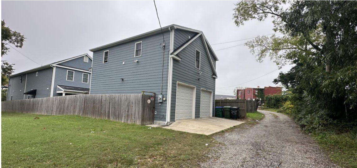
Figure 4: Picture of accessory building at 2413 Carrington fronting the rear alley
