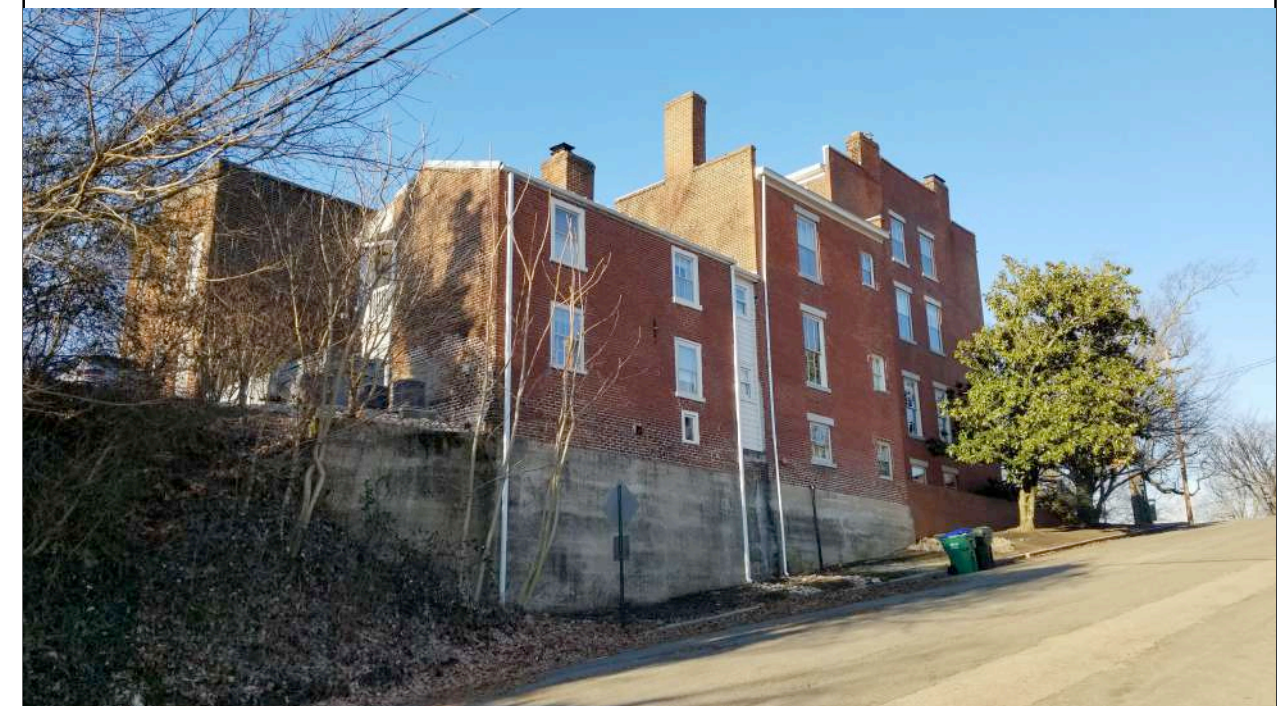
N 29TH ST. HOUSE ACROSS STREET
