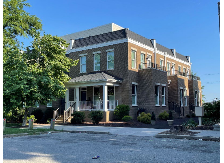
Figure 2. View of the south and east elevations of 1902-1908 Princess Anne Avenue. The proposed lighting will be secured to the building above the first-floor pairs of windows.
