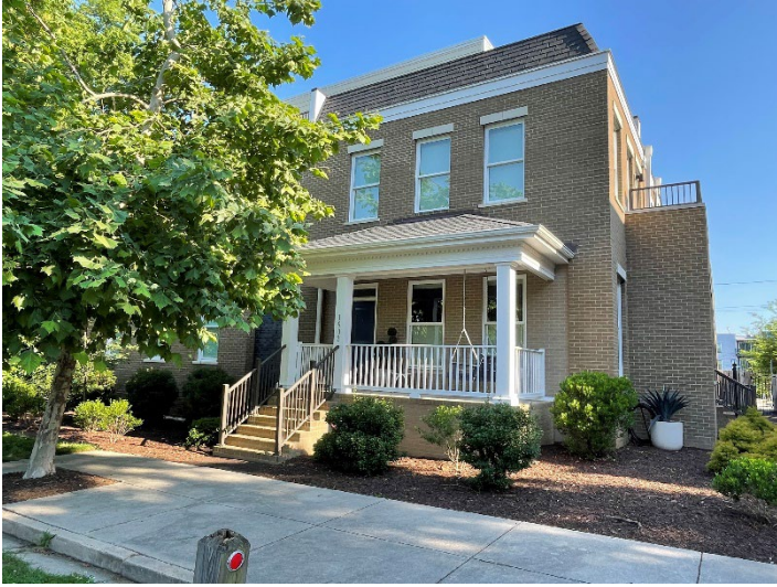
Figure 1. View of 1902-1908 Princess Anne Avenue's facade, at the west end of the dead-end street.
