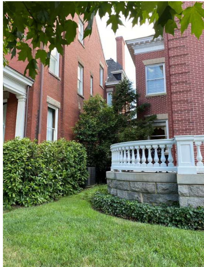
EXISTING FRONT VIEW
