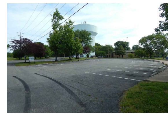
Existing Parking Lot Area to Receive Bioretention Basins
