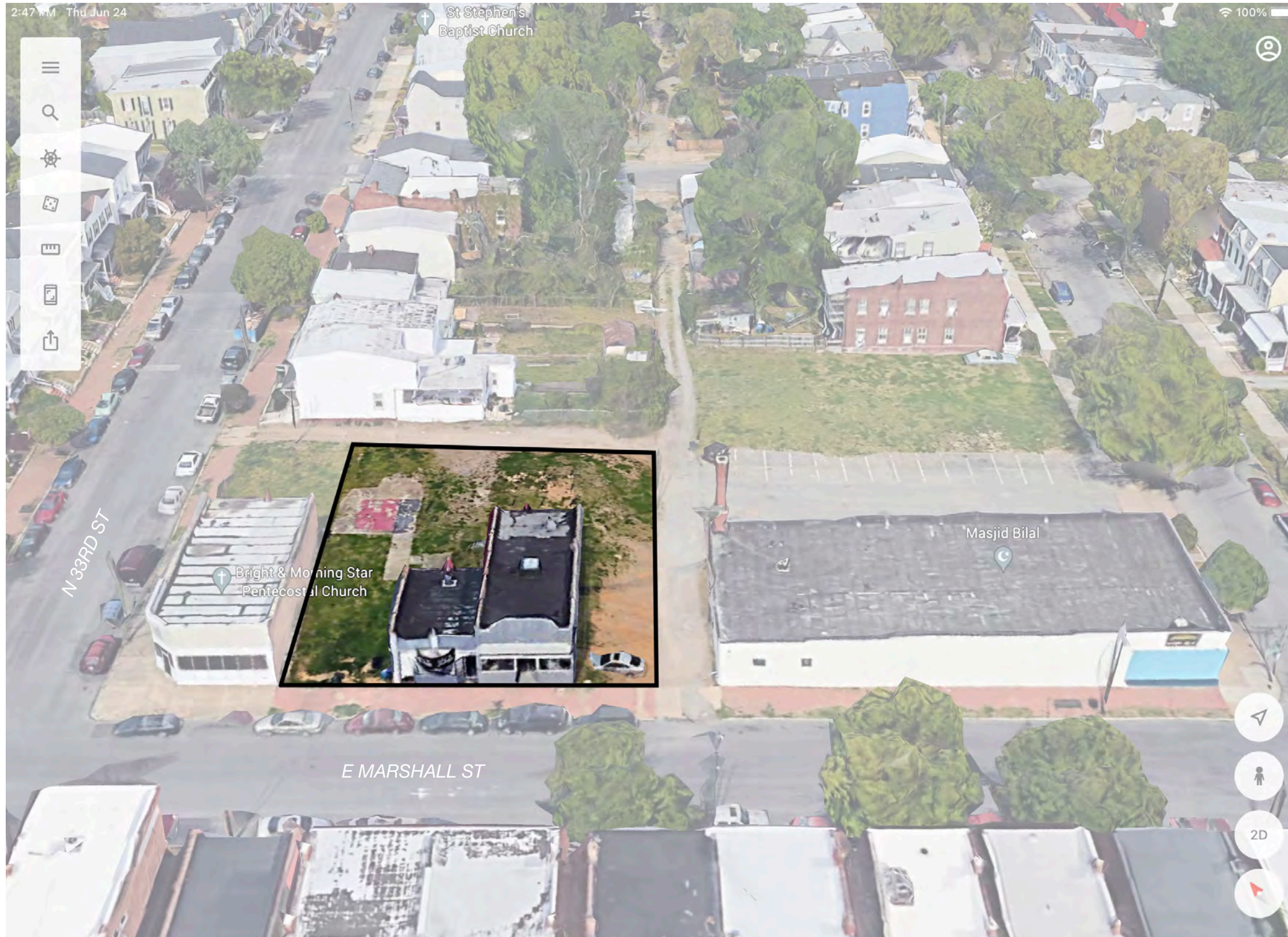
EXISTING CONTEXT - Showing existing buildings at 3304 and 3306 proposed to be removed.
