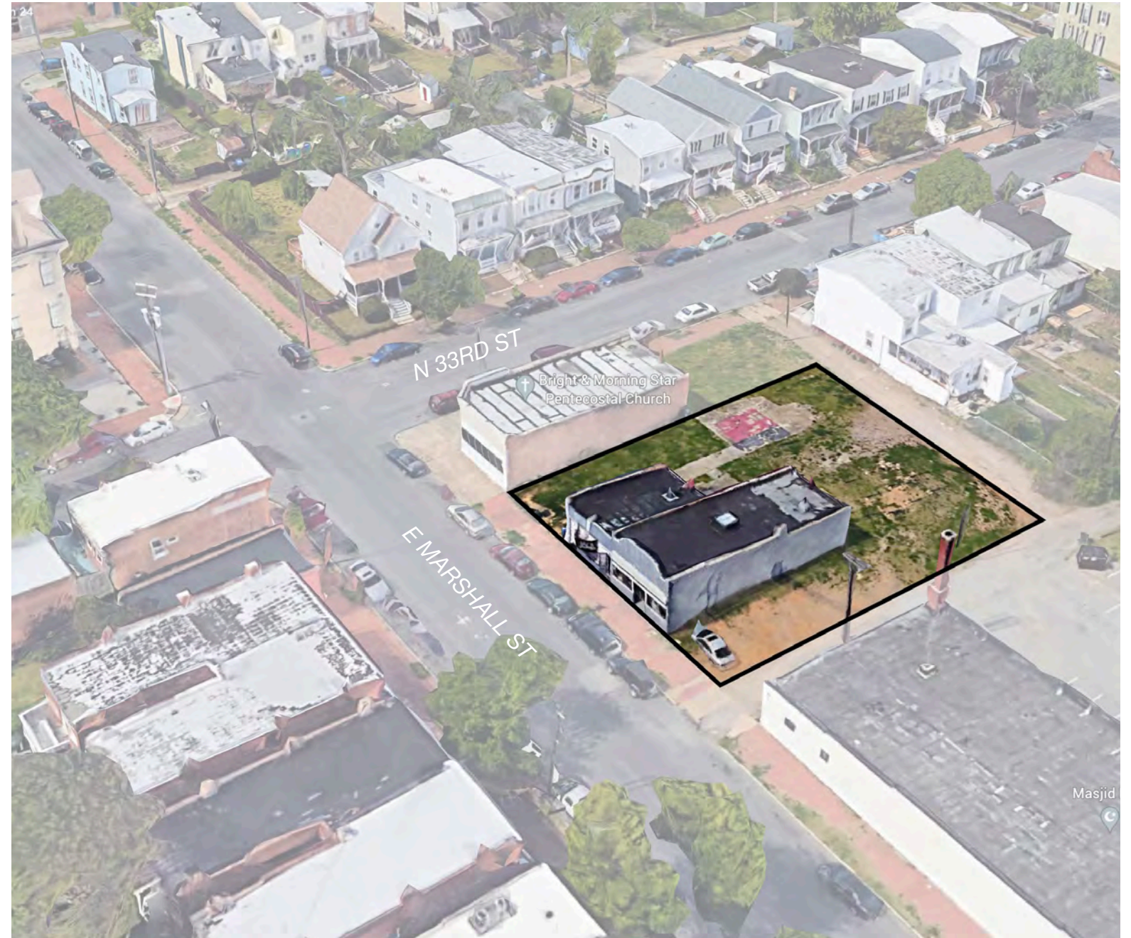
EXISTING CONTEXT - Showing existing buildings at 3304 and 3306 proposed to be removed. View from West View from East
