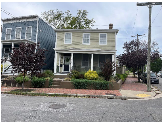
Figure 1. 2120 M Street Façade.
