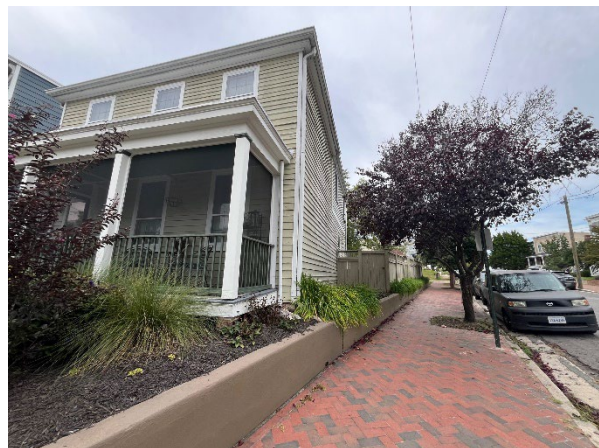
Figure 2. 2120 M Street, side elevation.
