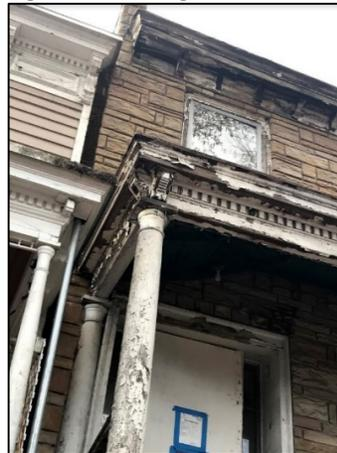
Figure 4. Column and Dental detail.
