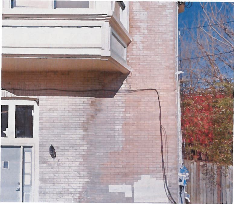
Staining on existing brick
