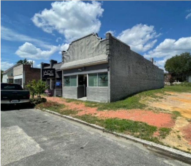
Figure 7. View of 3304-3306 East Marshall Street facades facing west.
