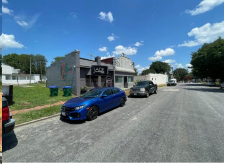
Figure 8. View of 3304-3306 East Marshall Street facades facing east.
