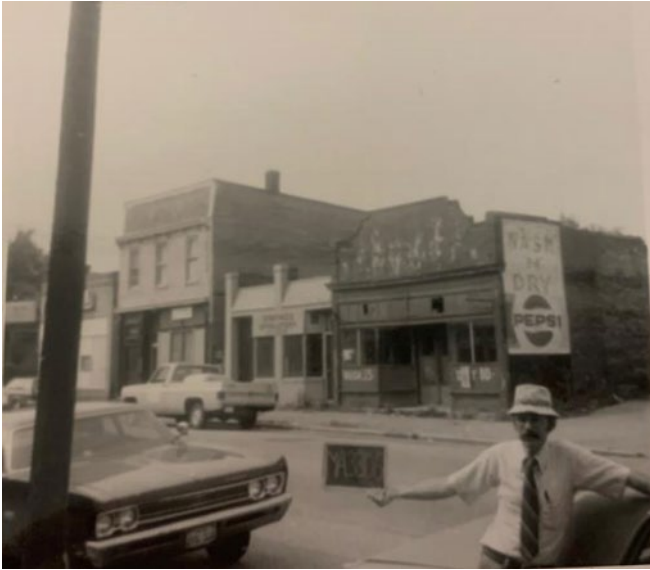
Figure 5. Historic photograph showing 3302-3306 East Marshall Street
