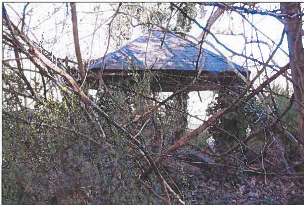
Photo 15: Early Twentieth-Century Gazebo/Tearoom, Looking North (Gordineer 2024).
