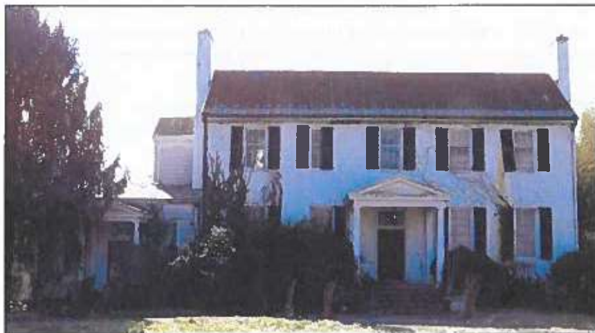
Photo 1: Brookbury, North Elevation (Gordineer 2024).
