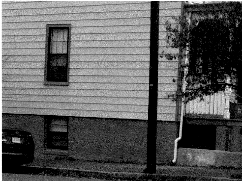
Another house in the Church Hill area with an English basement that has painted masonry and brick porch pillars
