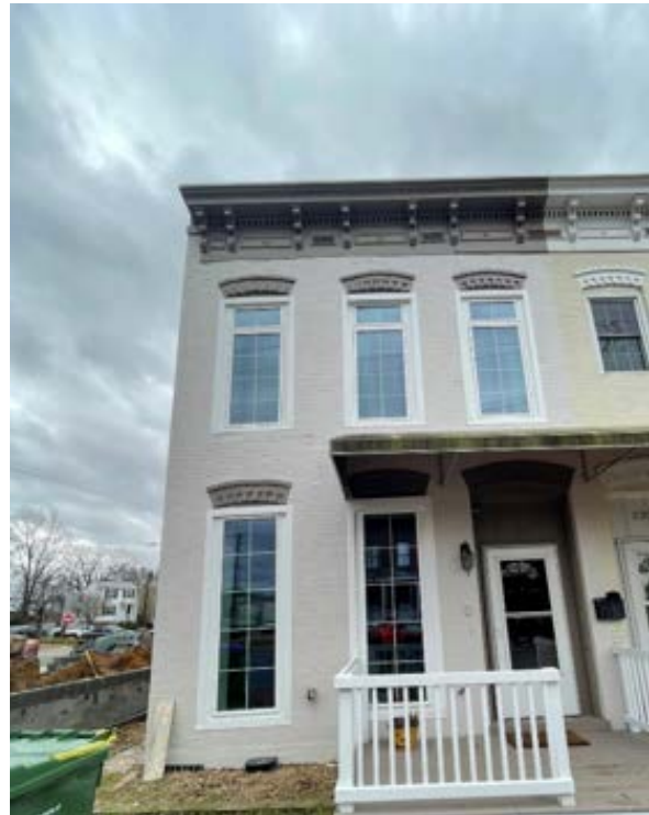
Figure 6. Front facade, 2323 Venable
