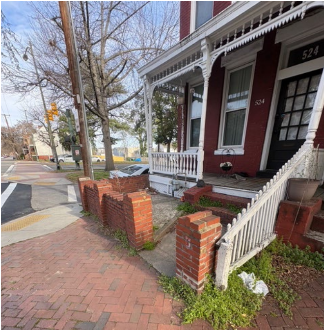
Figure 9. Brick Wall Example – Jackson Ward March 2026
