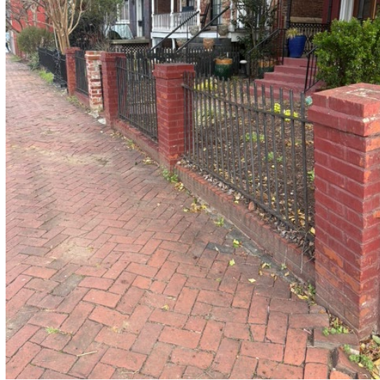
Figure 2. Brick Wall Example – Jackson Ward March 2026
