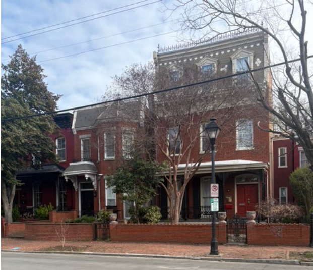
Figure 1. Brick Wall Example – Jackson Ward March 2026
