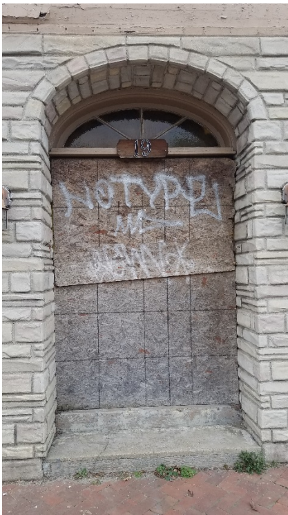
Figure 7. 19 W Leigh Street, door detail.
