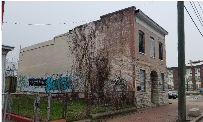
Figure 3. 19 W Leigh Street, south elevation.
