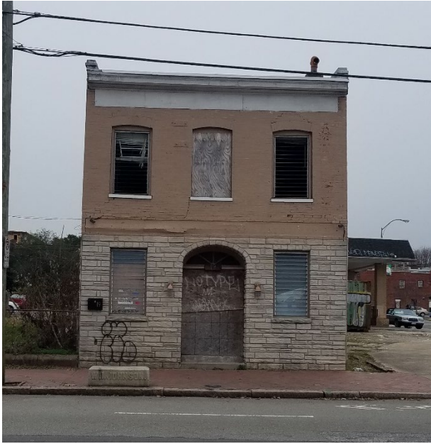
Figure 5. 19 W Leigh Street, facade.
