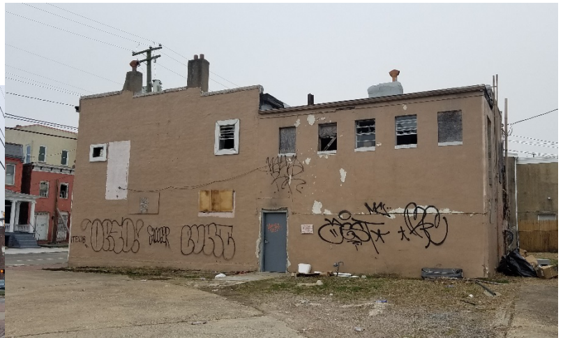
Figure 4. 19 W Leigh Street, north elevation.
