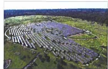
Montgomery County Oaks Landfill
