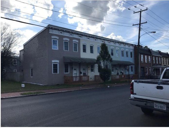
Figure 5. 2300 block Venable Street, odd side west of the subject lot
