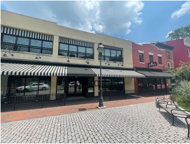
Figure 1. Existing conditions of 305-307 Brook Rd.
