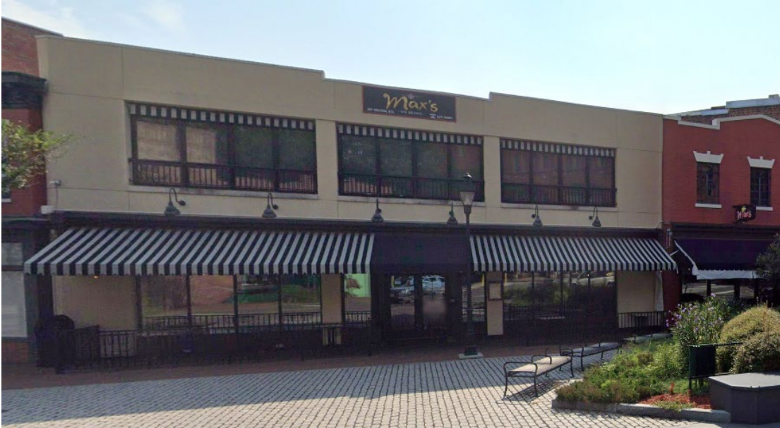
Figure 5. Original wall sign on 307 Brook Rd., removed
