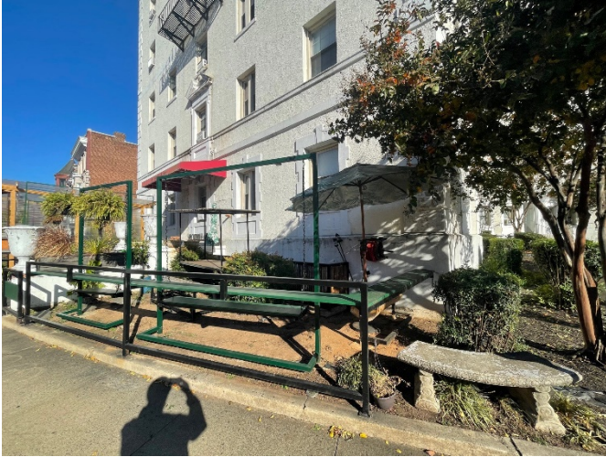
Figure 1. 1600 Monument Avenue. Existing Outdoor Seating. Tall green swinging seats will be removed.
