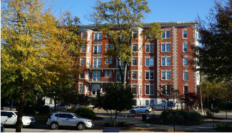
Figure 1. West, Primary Elevation
