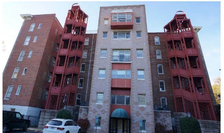
Figure 6. Rear, east elevation. Non-original stair towers, addition, and existing canopy.
