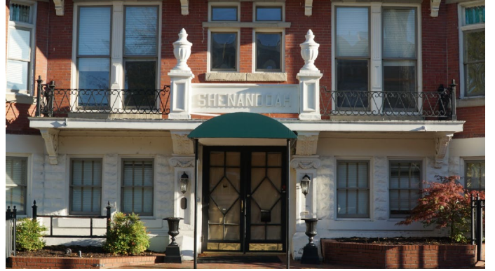
Figure 2. Primary entrance and existing canopy.
