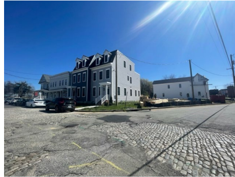
Figure 6. New construction at Carrington & Pink Streets
