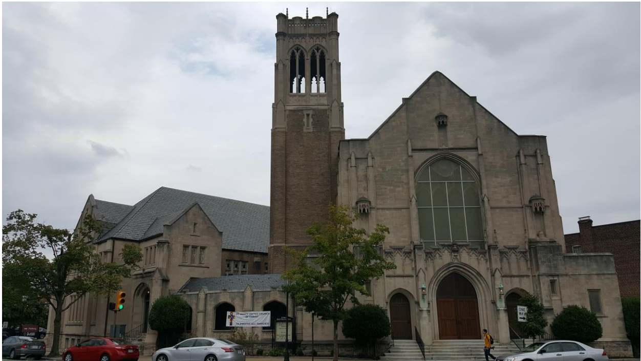
Adjacent property to the south across the alley, view from Stuart Circle
