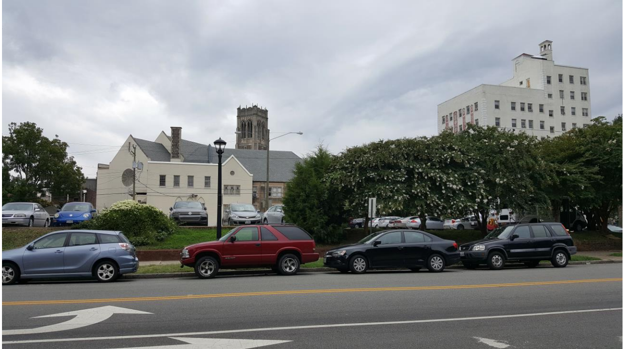
Subject property view from West Grace Street
