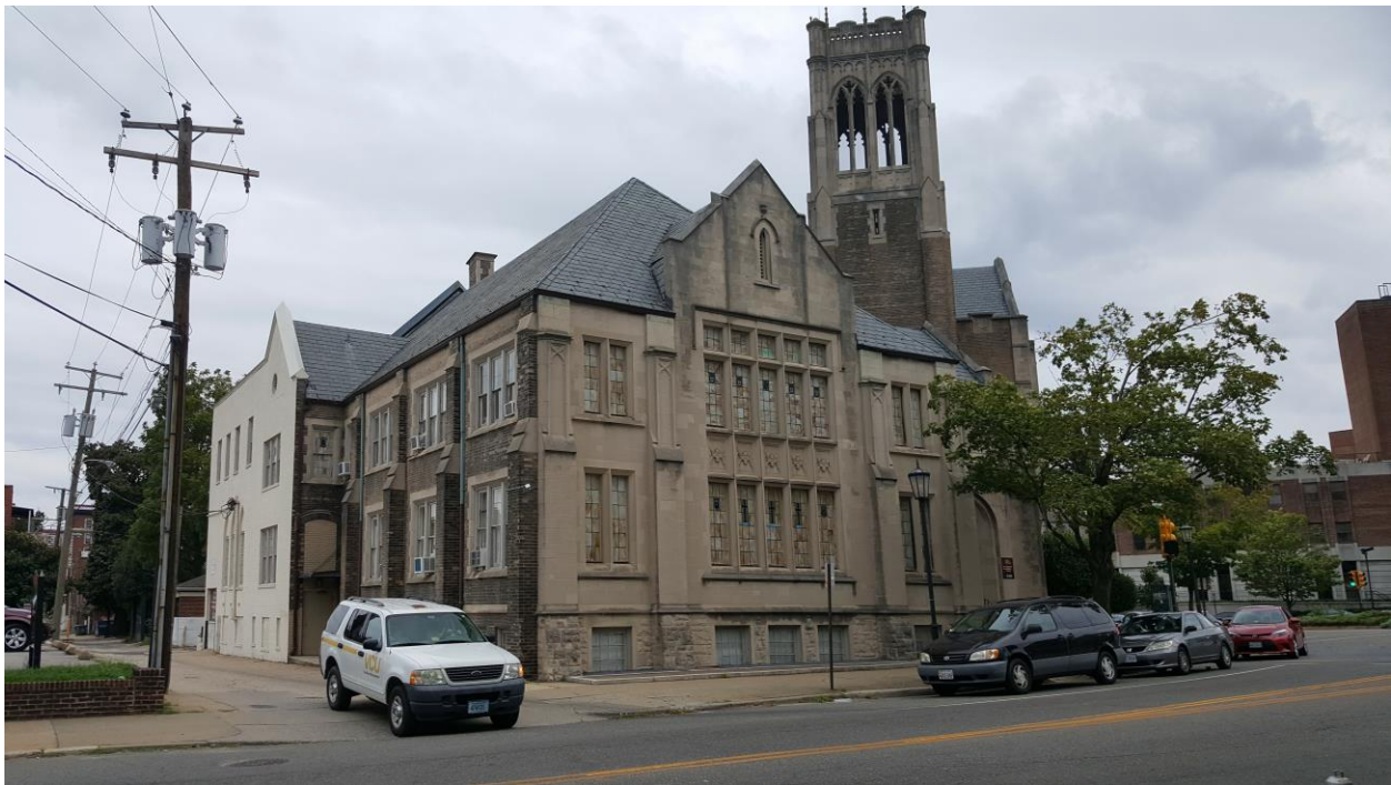
Adjacent property to the south across the alley, view from North Lombardy Street
