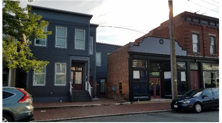
Figure 8. 3116-3118 East Marshall Street, mixed-use building with physical separation between the commercial and residential spaces.
