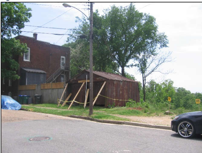
Figure 5. 130 North 32nd Street, garage
