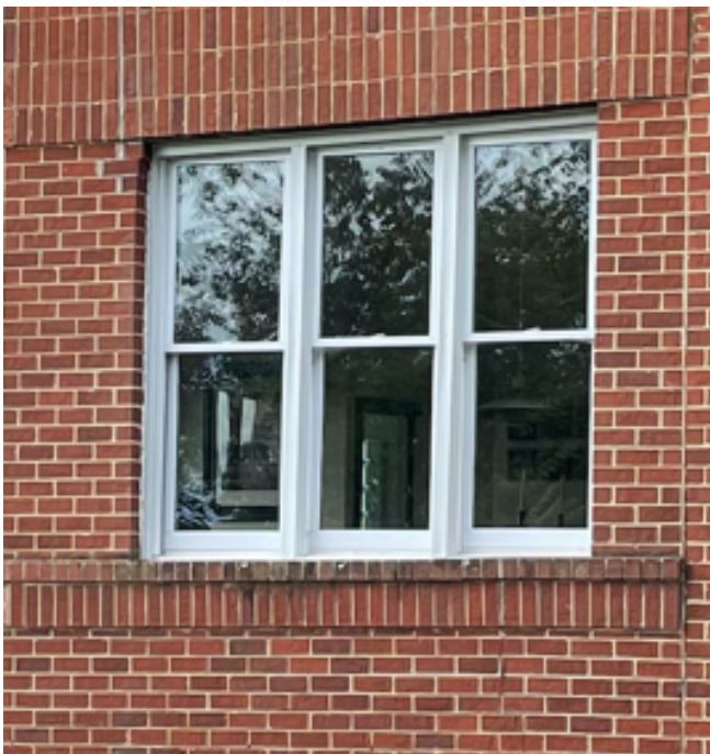
Damaged Bay Window & Brick
