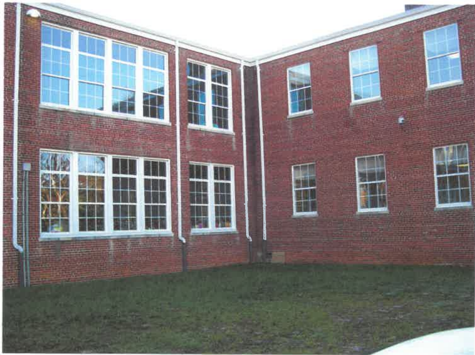
WEST WINDOW INSTALLATION at Campbell Court School Exterior 2
