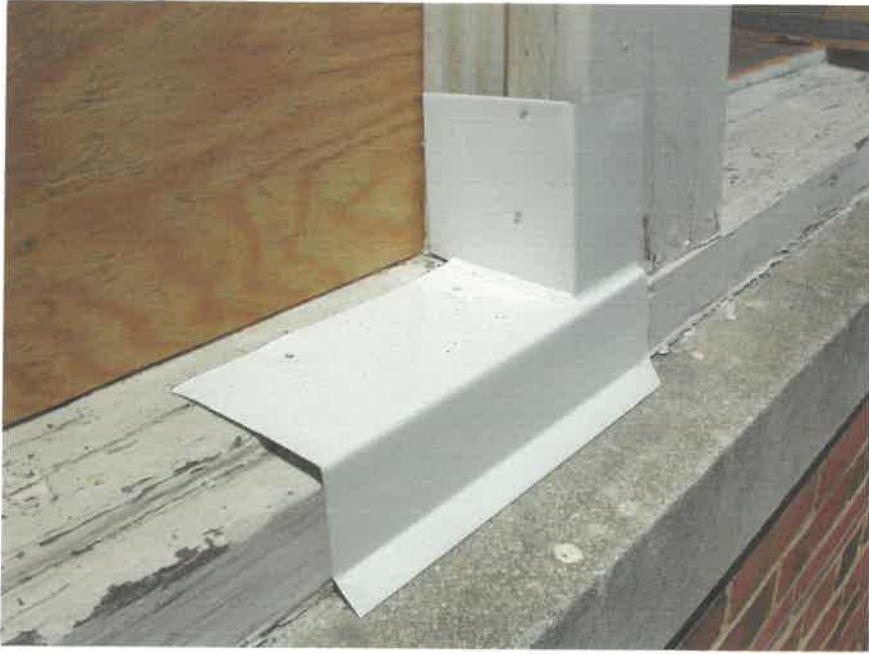
WEST WINDOW INSTALLATION at Campbell Court School Bottom Wrap 1
