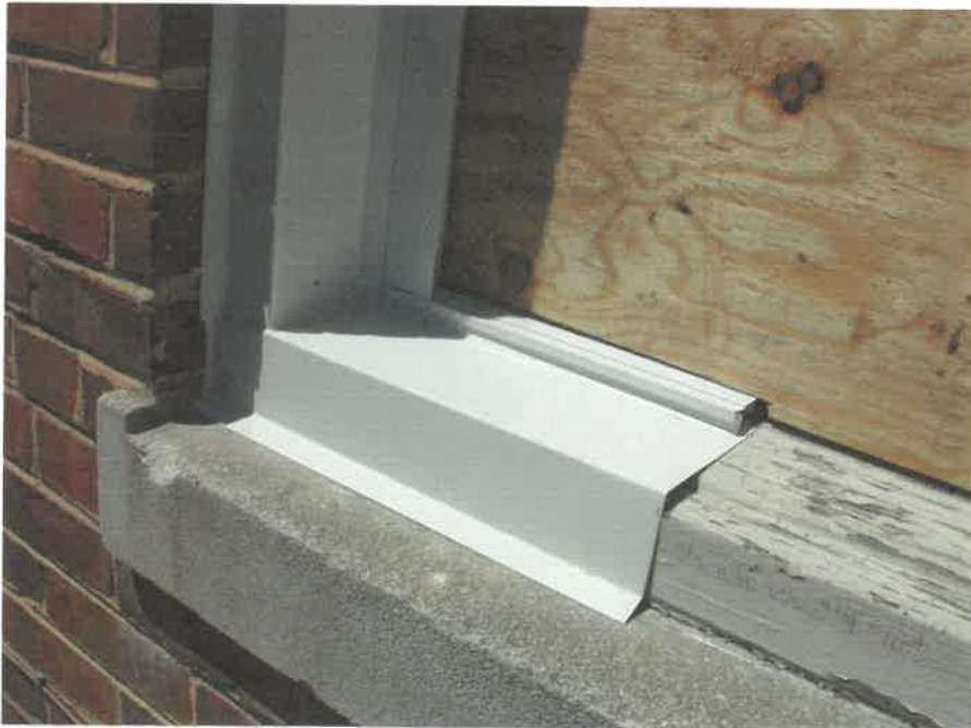
WEST WINDOW INSTALLATION at Campbell Court School Bottom Wrap 2
