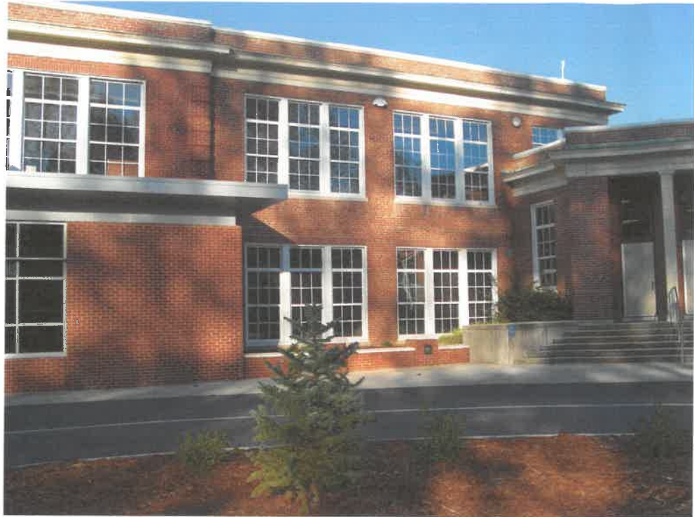
WEST WINDOW INSTALLATION at Campbell Court School Exterior 1
