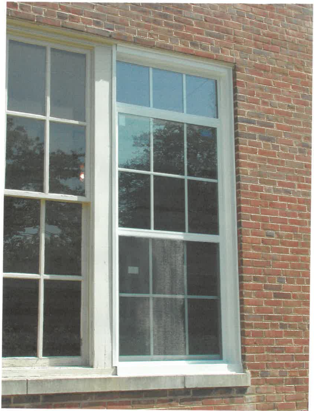
WEST WINDOW INSTALLATION at Campbell Court School Old and New
