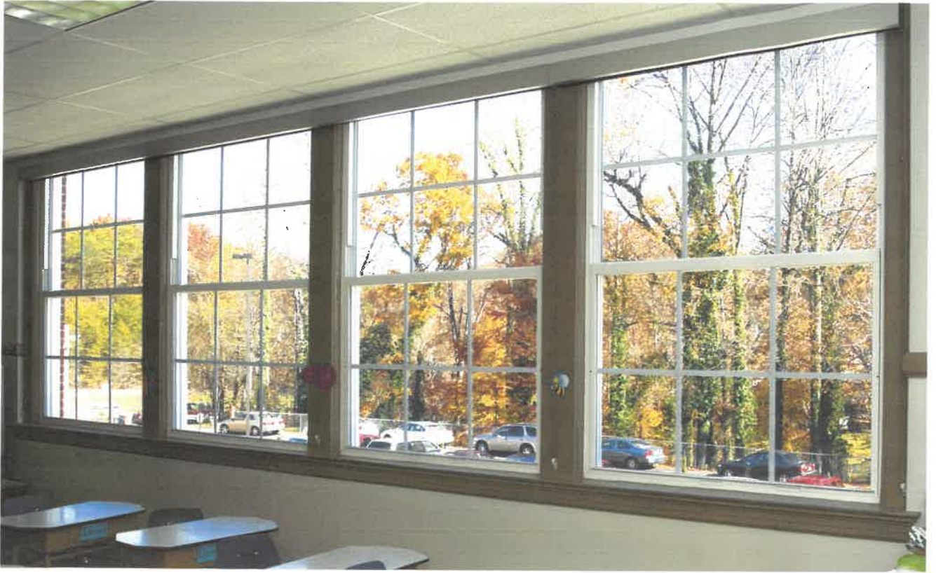
WEST WINDOW INSTALLATION at Campbell Court School Interior 3
