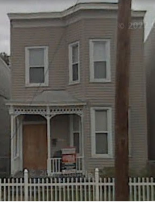
Figure 1. Image of original front porch (2007) with circle motifs in the frieze. Sawn pickets appear to have been removed by this time. Google street view, accessed 7/12/2023
