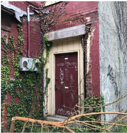
Figure 5. Existing front entrance
