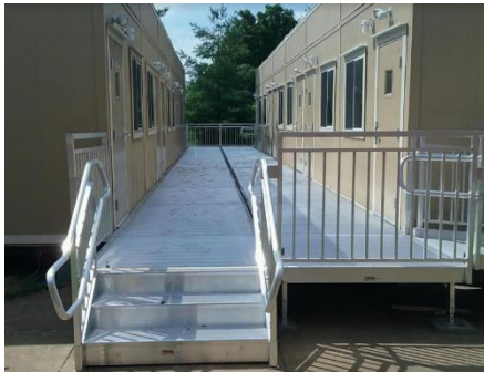
Typical Lease Metal Deckin/Stairs
