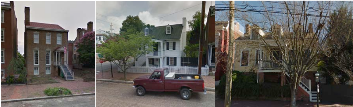
Second floor entry stairs – 2302 & 2500 E Grace St & 207 N 25 th Street
