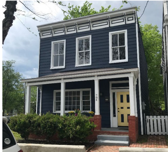
Figure 2. 704 North 24th Street, façade
