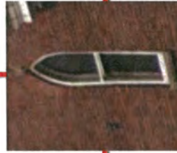
TRANSPARENT GLASS IN BOTTOM PORTION OF WINDOW STAIN GLASS TO REMAIN AT TOP PORTION OF WINDOWS. COLORS WILL MATCH EXISTING STAIN GLASS WINDOW COLOR VARIATIONS.
