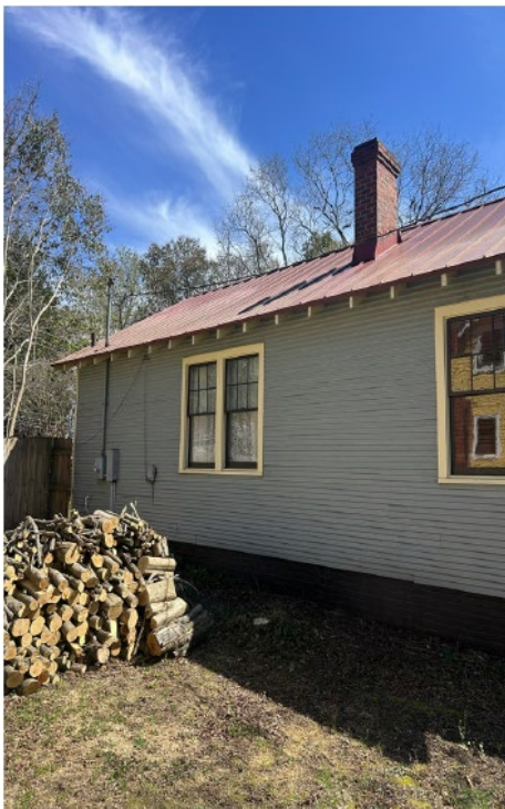
Figure 3: Northwest Elevation of the rear side of 517 W 21 st St
