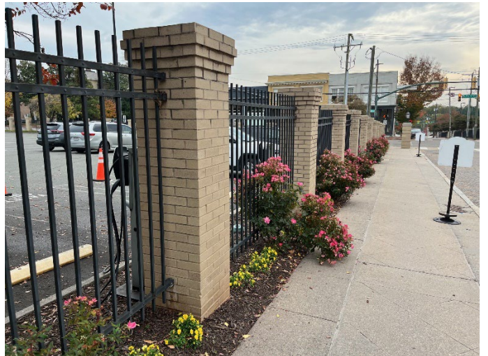
Figure 4. Existing fence. Brick piers and metal fencing. To be replication adjacent to demolished Valet Building.
