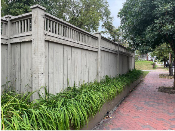
Figure 5. The existing privacy fence to be extended.
