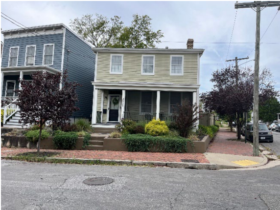
Figure 1. 2120 M Street Façade.
