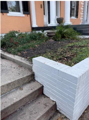
Figure 3. Cement retaining wall connection to the existing masonry wall.
