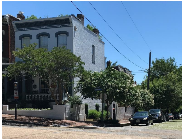
Figure 4. Brick wall at East Grace and North 26th Streets.
