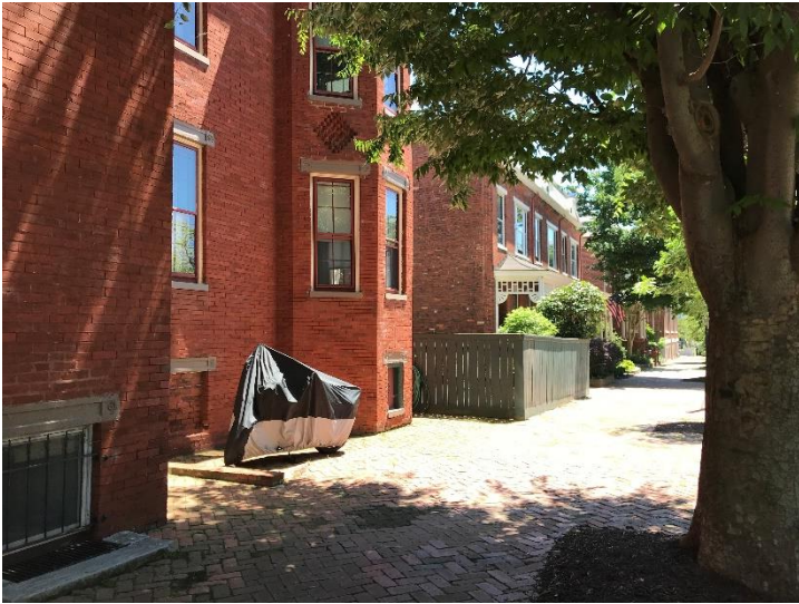
Figure 1. 2601 East Broad Street, corner elevation.
