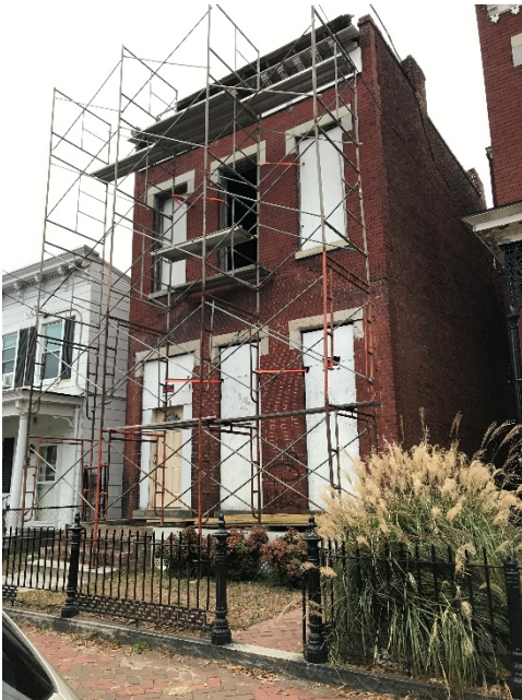
Figure 3. 416 West Clay Street, existing conditions.
