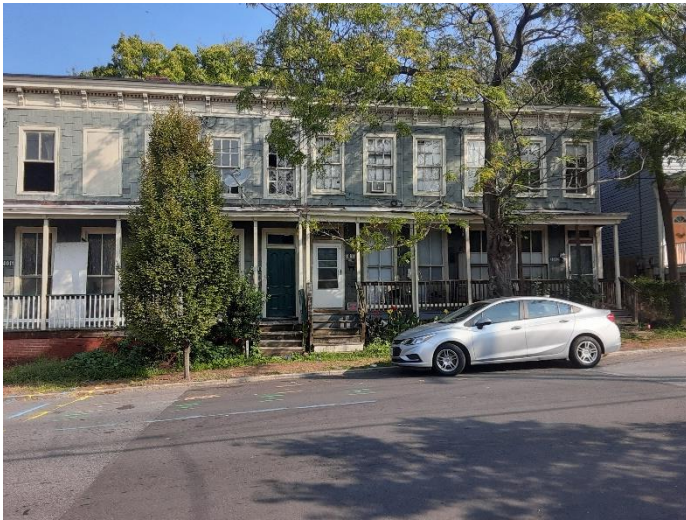
Figure 1. 2010-2012 Venable Street, façade
