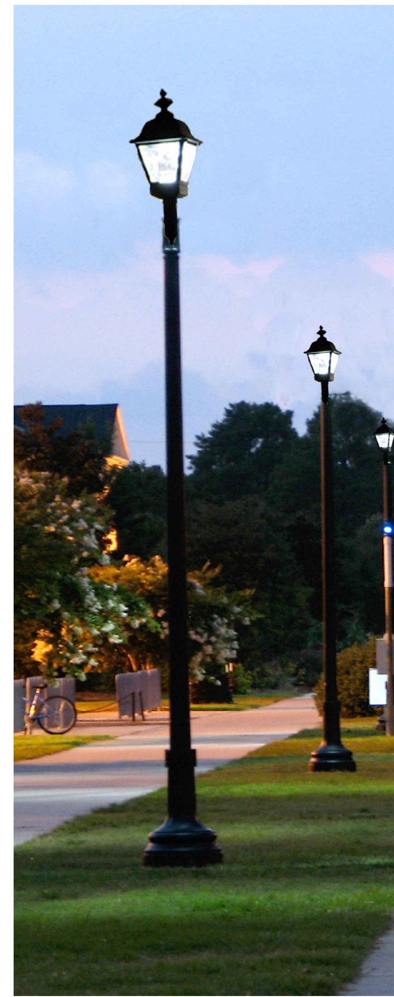
LIGHT POLE & POLE PHOTO NO SCALE
