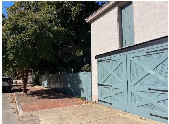
Figure 4. Rear carriage house and privacy fence located at 2720 E. Broad Street.
