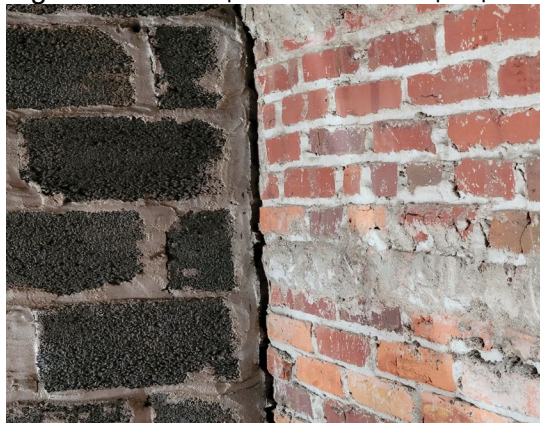
Figure 4. Wall separation and improper repairs.
