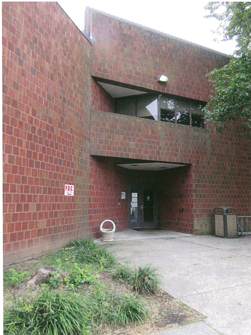
EDI BUILDING 701 NORTH 25TH STREET RICHMOND, VIRGINIA 23230
