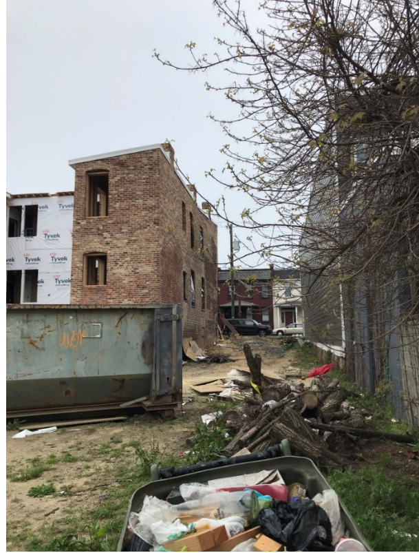
Figure 2. View of lot from rear alley
