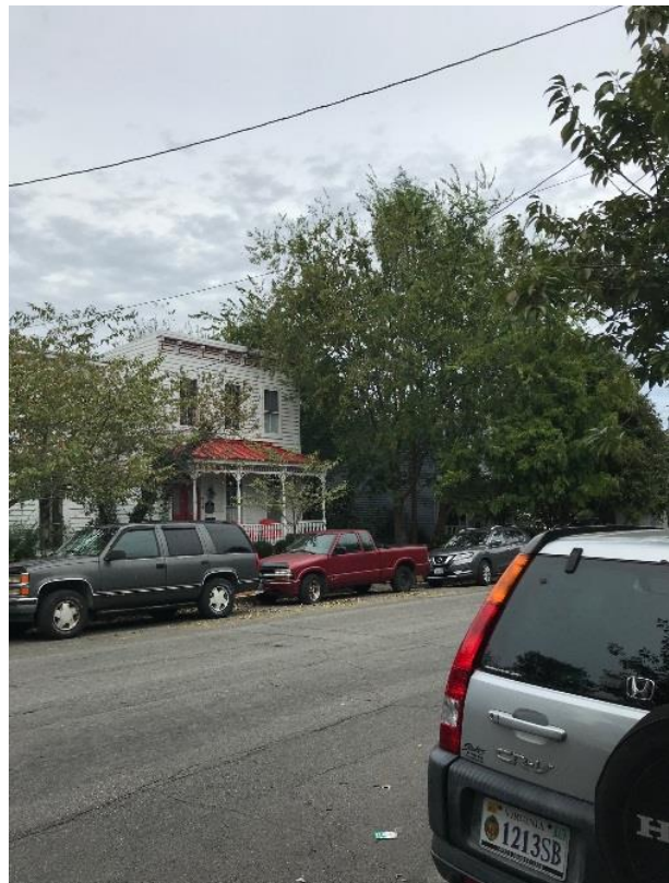
Photograph 2. 418 North 23rd Street, current conditions.
