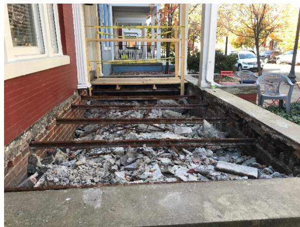
Figure 4. 2609 W. Grace Street Front Porch Floor Removed
