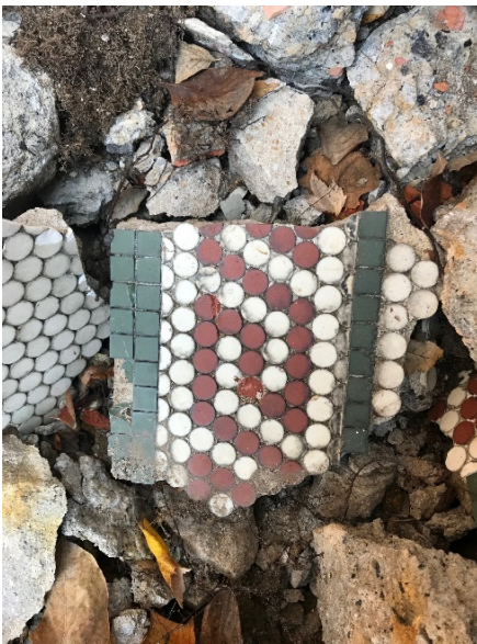
Figure 3. Remnants of Original Tile Removed from Porch Floor
