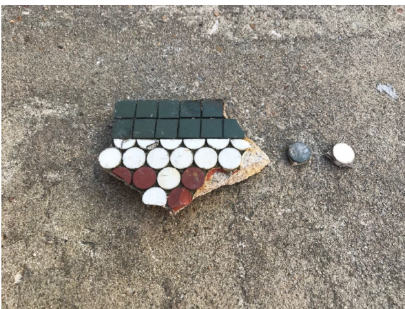
Figure 5. Remnants of Original Tile Removed from Porch Floor
