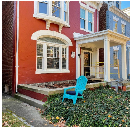
Figure 2. 2609 W. Grace Street Front Porch Floor Removed
