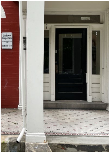
Figure 1. 2609 W. Grace Original Front Porch Floor
