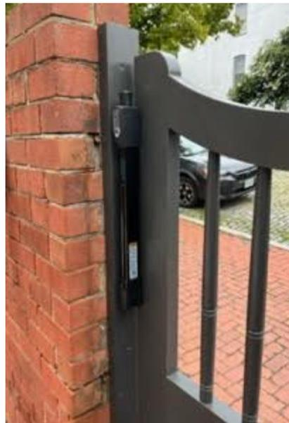
Images 24-25: Back gate in alley – view from East 26<sup>th</sup> Street looking north. Code compliant latch that cannot be viewed from the outside.
