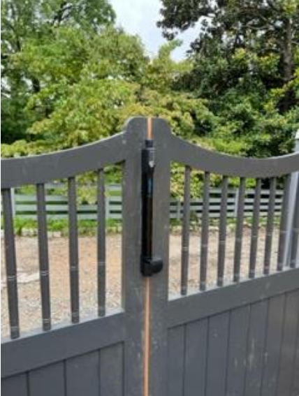
Images 24-25: Back gate in alley – view from East 26 th Street looking north. Code compliant latch that cannot be viewed from the outside.
