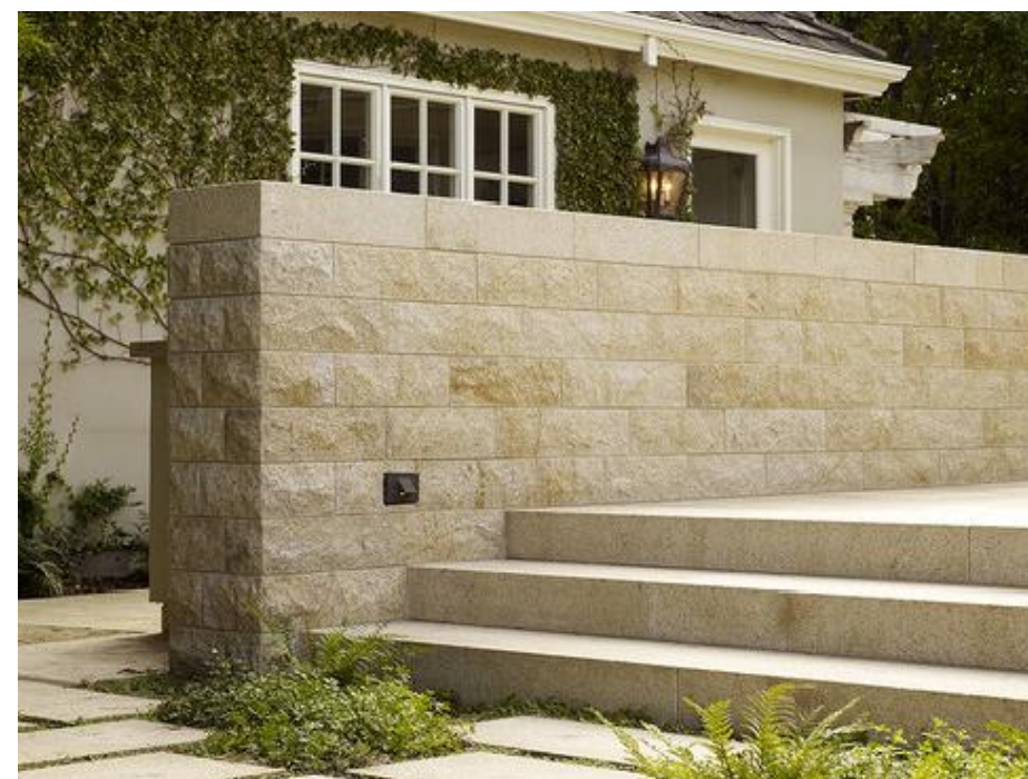
LIMESTONE STAIR TREADS (12"x72"x2") (STRAIGHT EDGE) POSSIBLE SOURCE: INDIANA LIMESTONE FULL COLOR BLEND (SHADE & WISE)
