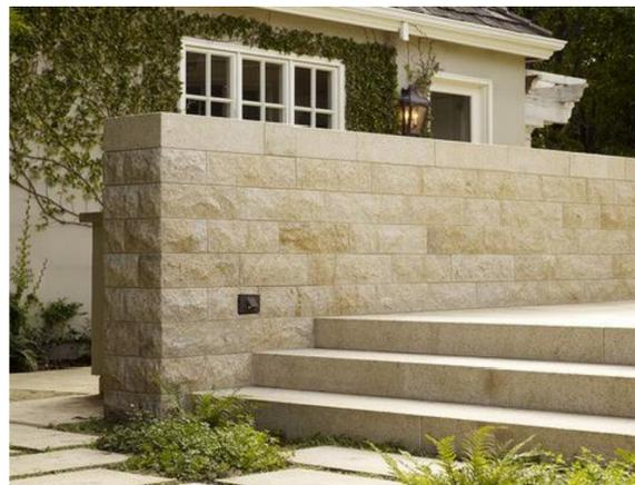
LIMESTONE WALL BLOCK (6"H) WITH LIMESTONE CAP (SMOOTH EDGE FINISH)
