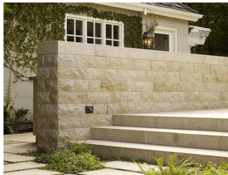
LIMESTONE WALL BLOCK (6"H) WITH LIMESTONE CAP (SMOOTH EDGE FINISH) POSSIBLE SOURCE: INDIANA LIMESTONE FULL COLOR BLEND (SHADE & WISE)
