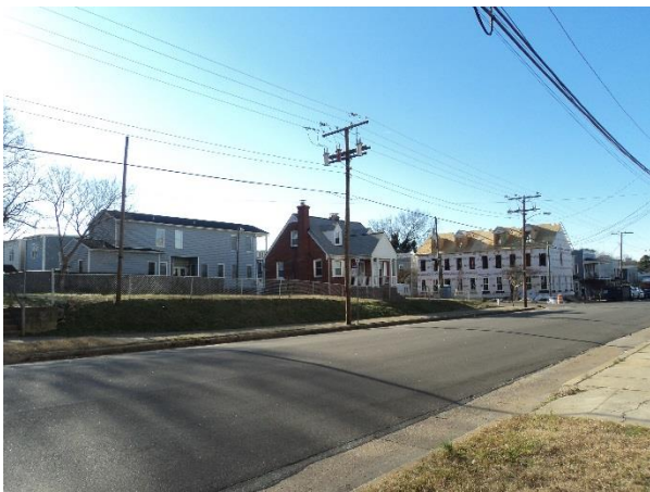
Figure 5. 2901 M Street with view of new construction.
