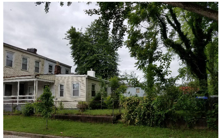
Figure 6. View to rear from Jessamine Street.
