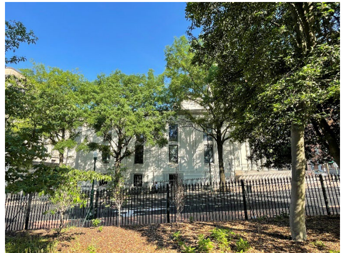
Figure 8. View of the Church's east elevation from Capital Square. This elevation will likely be more visible in the fall.
