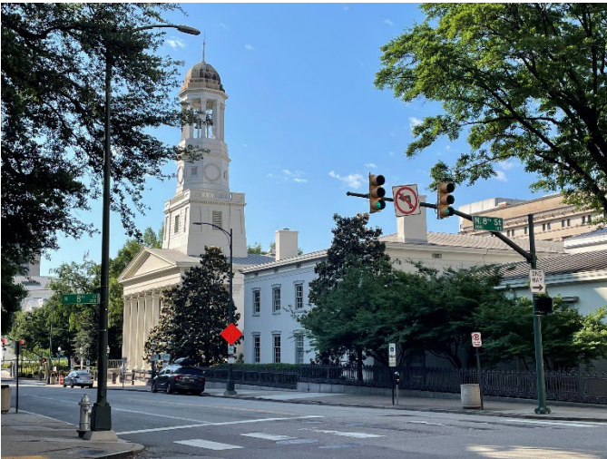
Figure 3. West elevation of St. Paul's Episcopal Church. The applicant proposes installing solar panels on west and east sides of the historic roof, south of the bell tower and north of the projecting bay on the rear.
