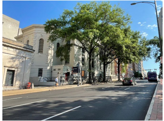
Figure 6. View of the rear, south elevation of the Church.
